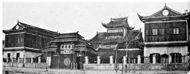
The Imperial Maritime Customs House (first building)
